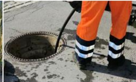
Sewer flooding (Anglian Water , Thames Water)
