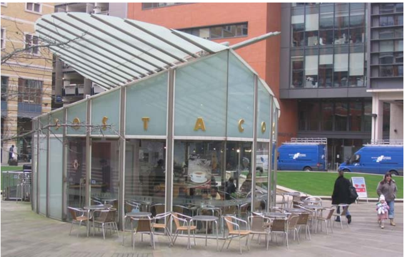
A cafe pavillion as an architectural centrepoin
