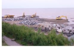
core material is placed by excavators and covered by a geotextile to form the middle of the structure.
