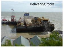
and brought to the beach at around high water and deposited, near to where each groyne is to be constructed. The rocks are then moved into place by land-based machinery.
