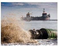
The "Causeway" will deliver beach material up to four times a day. It will place approximately 62,500 m³ of material a week, which will fill up one bay.
