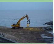
All timber and concrete groynes and the wave dissipation structures have now been removed.
