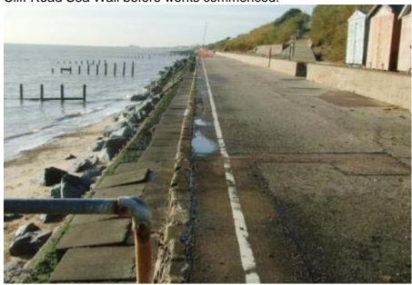
The scheme location was between Fernwood Avenue and Cliff Road and the site compound was located in the Brighton Road car park. The scheme consisted of 230m of sea wall supported by rock armour, a concrete vehicular access ramp and a set of timber steps.
