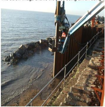
The below image shows the completed access ramp piling
