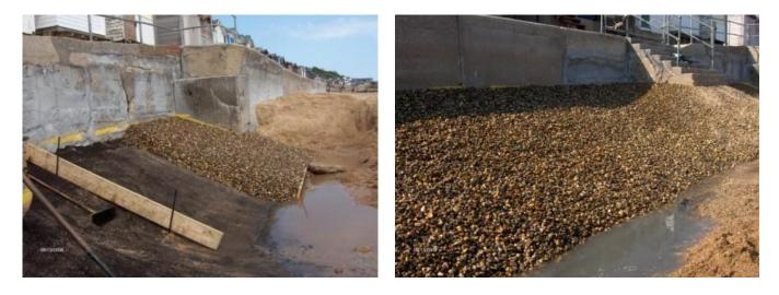
Approximately 130 metres of the seawall has now been treated where serious erosion often occurs during the severe winter storms. The reinforcing consists of forming a 3 metre wide wedge of Elastocoast material below normal beach level to seal the lowest section of the seawall against undermining by storm tides.
