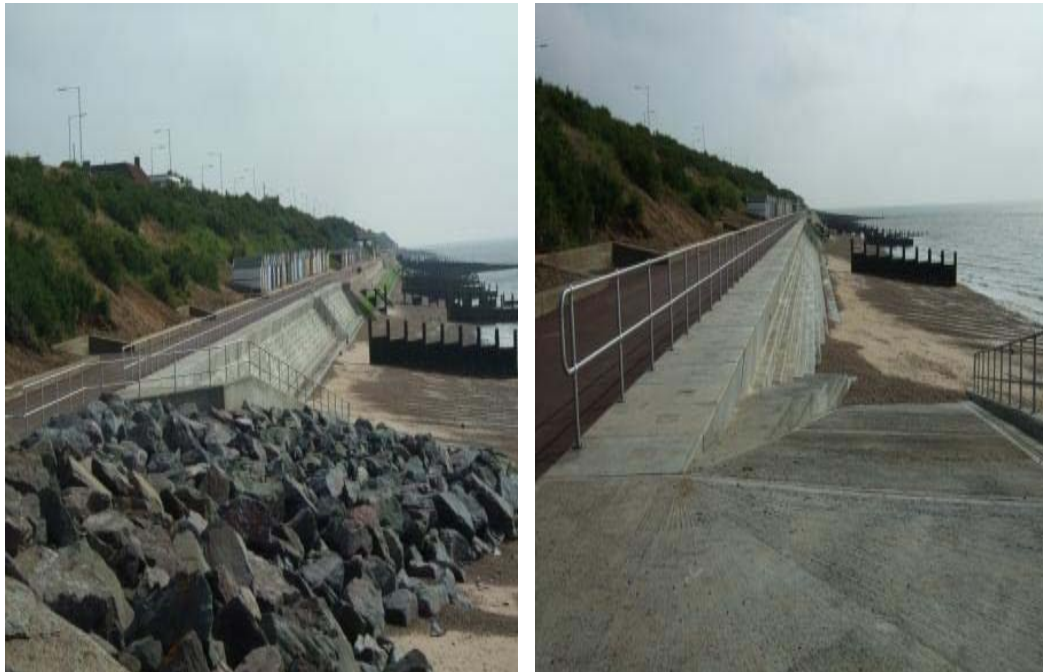
Completed works (June 2009)
