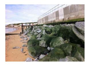
The work consisted of removing a section of the corroding sheet pile at the top of the structure and replacing it with new precast concrete units. Also included was a new piled toe together with protective rock armour to support the existing structure. The length of seawall that has been improved is approximately 80 metres.
