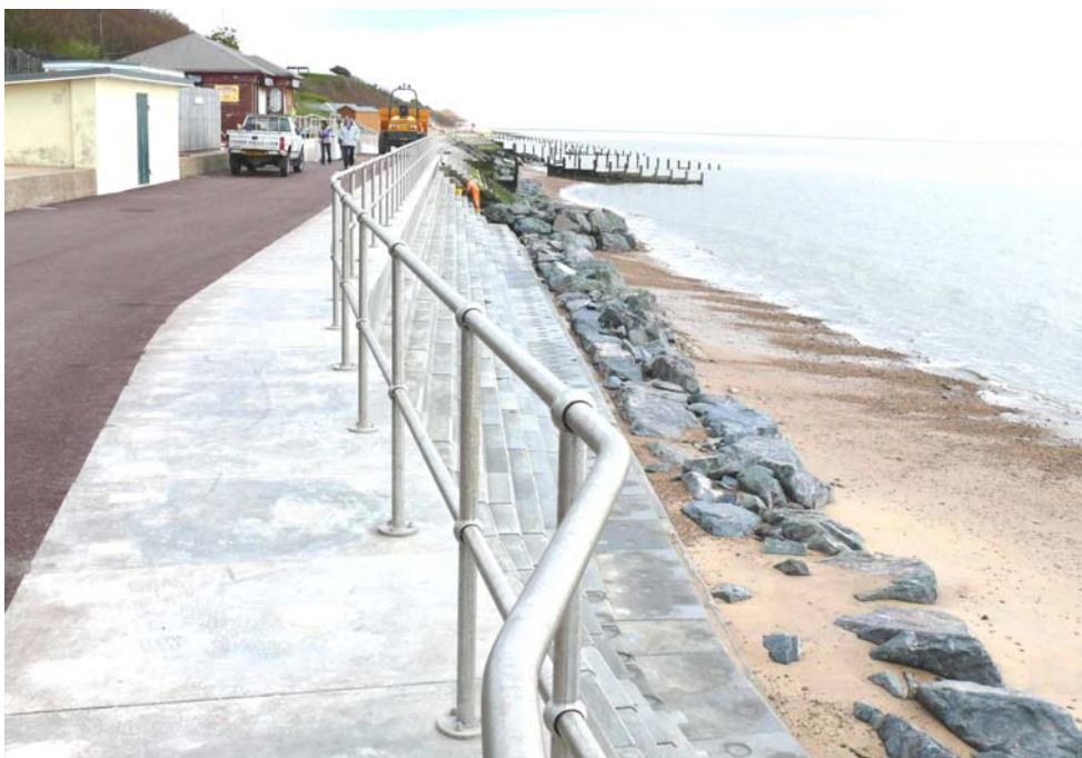
Completed works (May 2010)
