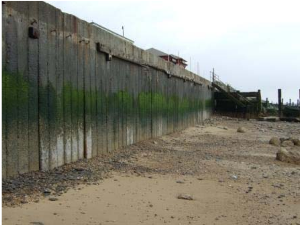
York Road seawall before works commenced.
