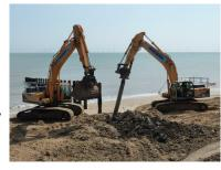
The beaches will initially be recharged with sand and shingle taken from a Crown Estates licensed site approximately 19kms offshore, in order to raise the levels where the new groynes are to be constructed.
