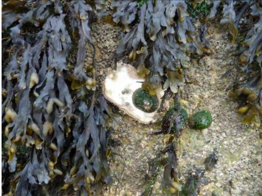
Brown sea weed growing on a concrete groyne
