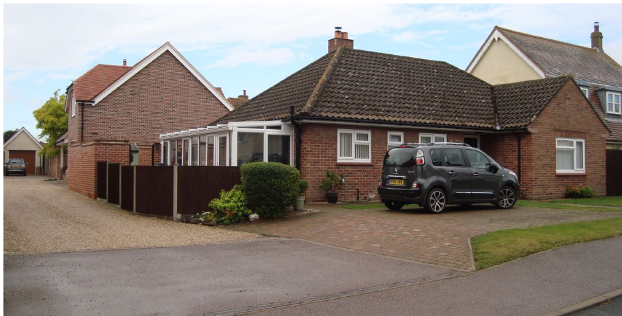
Figure 55 Post-war bungalows are an untraditional building type for the Conservation Area
