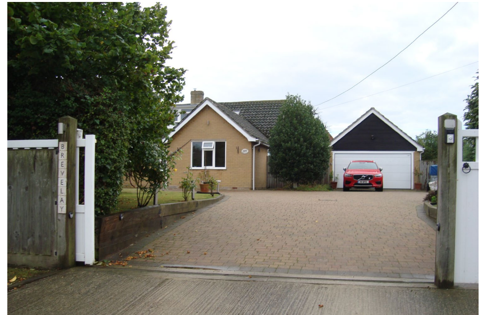
Figure 47 Inappropriate materials including yellow brick and concrete tiles on modern dwellings
