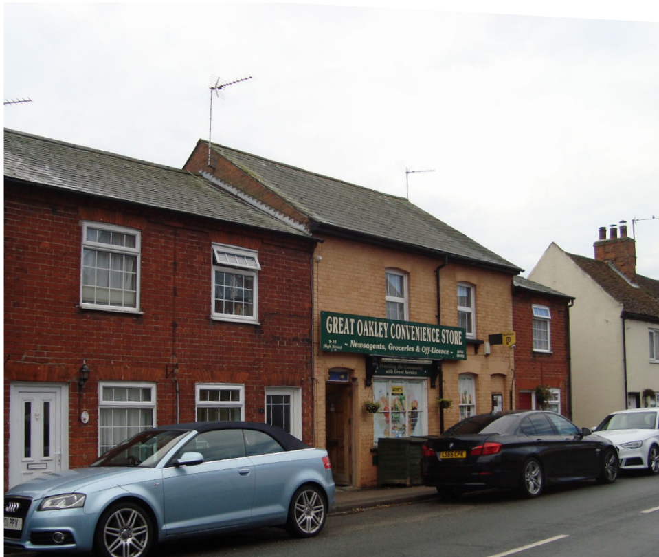
Figure 57 Convenience store on High Street
