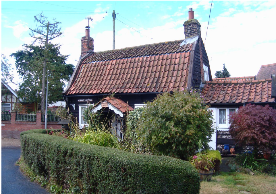
Figure 30 Grade II listed Florence Cottage with weatherboarded walls, clay pantile gambrel roof and boundary hedge
