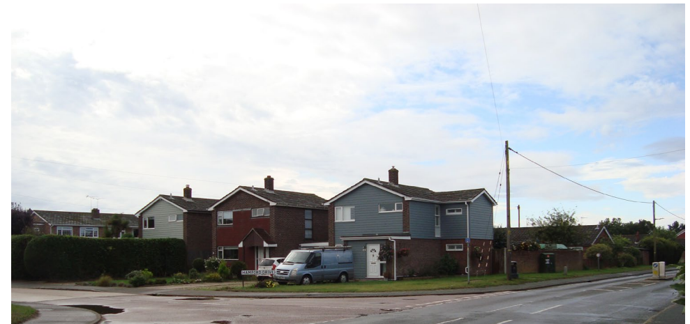
Figure 43 Post-war housing along Hamford Drive forms the setting of the Conservation Area to the west
