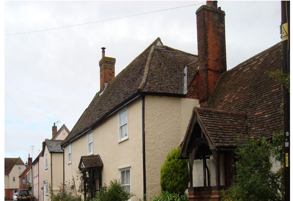
Figure 31 Grade II listed Maltings Farmhouse, a timber-framed and roughcast rendered house with fifteenth-century origins
