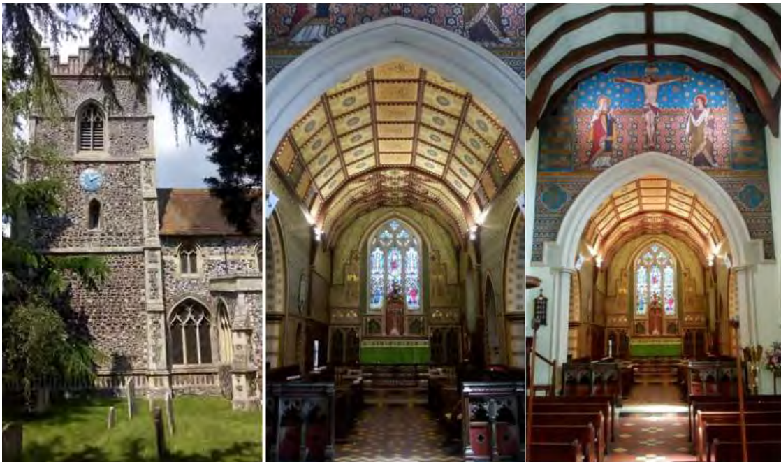
Fig. 19. The Grade II* listed St Mary's Church
