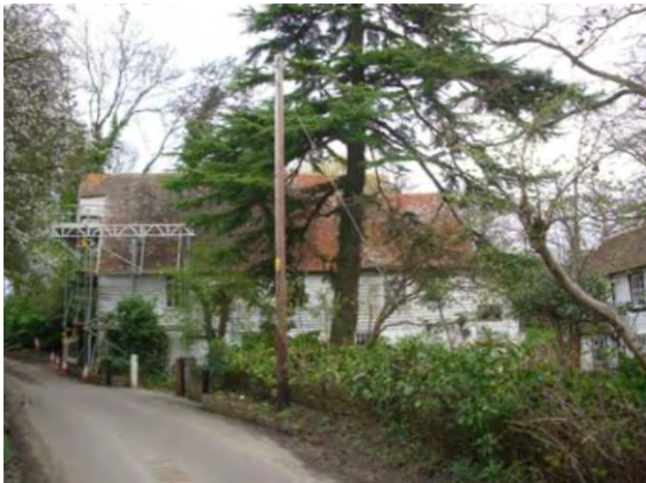
Fig. 21. The Grade II* listed Spring Valley Mill
