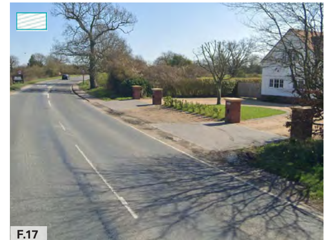
Figure 17: Individual house set within the countryside.
