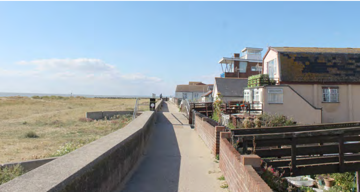
Fig. C31. View of Brooklands seafront (DU2) - current condition.
