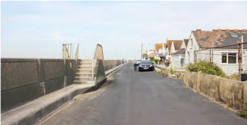
Fig. 75. Photograph of current condition of Brooklands.
