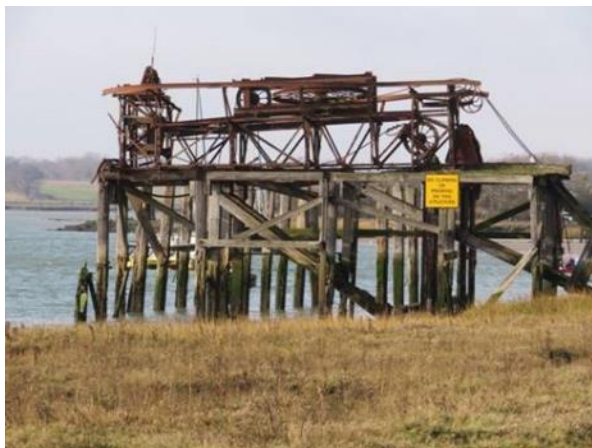
Ballast barge jetty and bucket chain pylon gravel conveyor system, Alresford Creek
