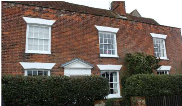
Figure 70 Grade II Listed 42 Queen Street
