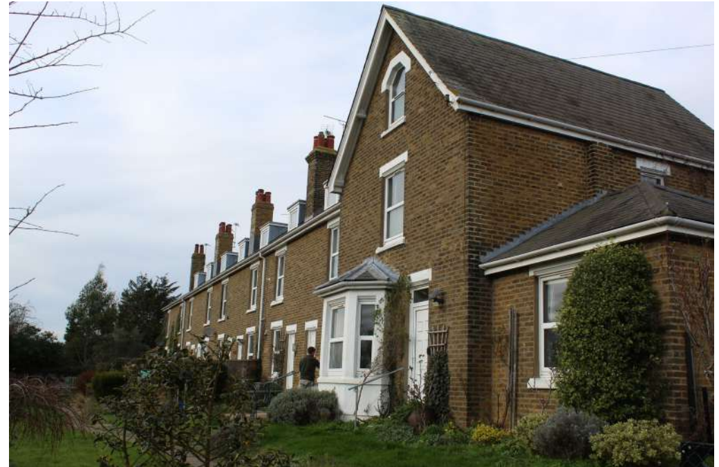
Figure 37 Florence Cottages, Back Waterside Lane
