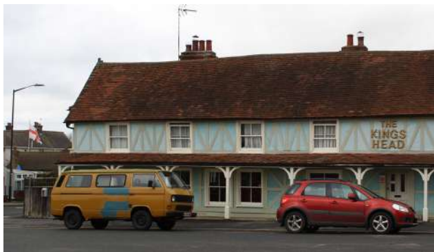
Figure 66 Grade II Listed Kings Head
