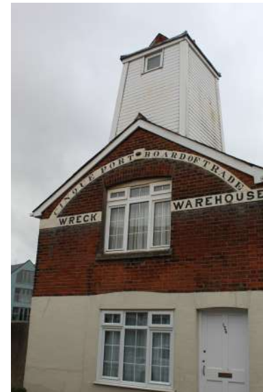
Figure 47 Wreck Warehouse Sydney Street
