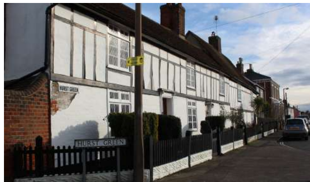
Figure 27 Grade II Listed 29 and 30 Hurst Green
