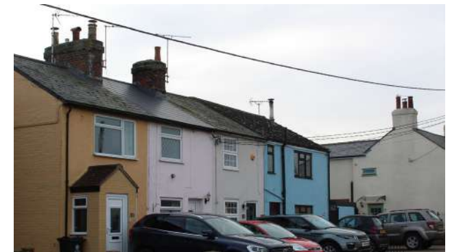
Figure 28 Buildings on Mill Street
