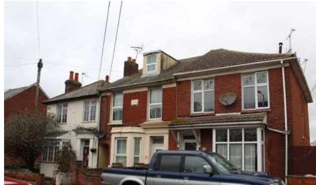
Figure 58 Example of terracing on Station Road
