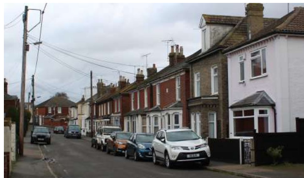
Figure 53 View of terraced housing
