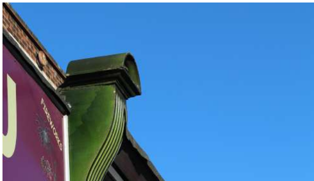
Figure 31 Green tiled console at the top of a pilaster
