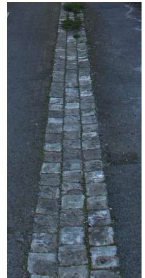
Figure 36 Scoria bricks on Crown Lane
