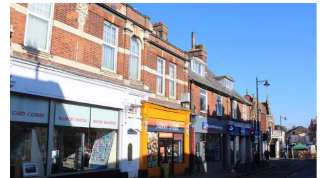
Figure 30 Shopfronts on the High Street
