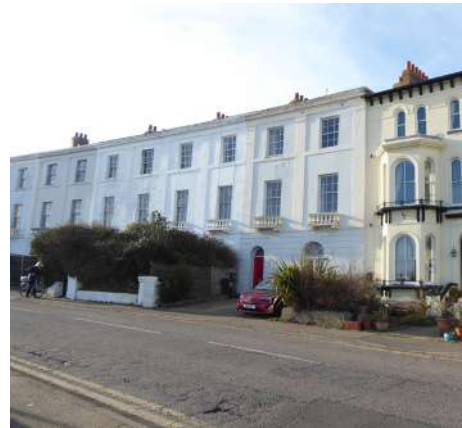
Figure 62 Three storey terraced row
