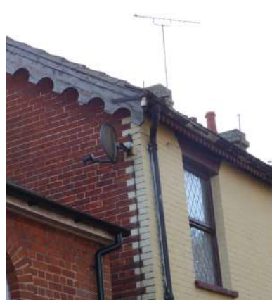
Figure 73 Decorative eaves and corner brick detail
