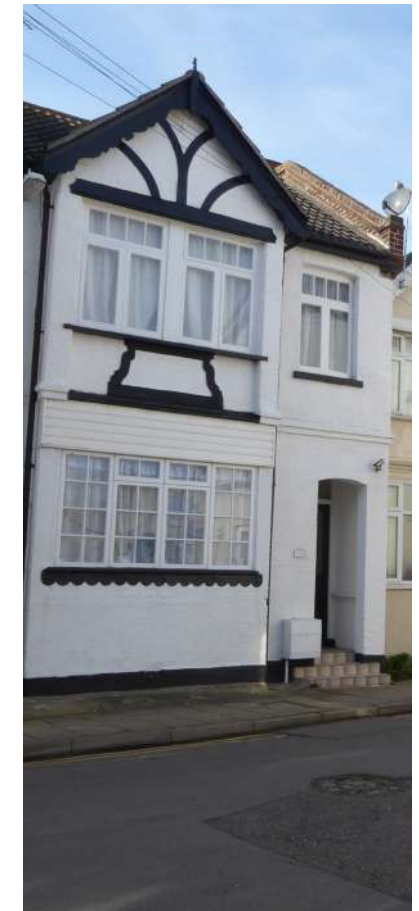
Figure 72 Number 13 New Pier Street
