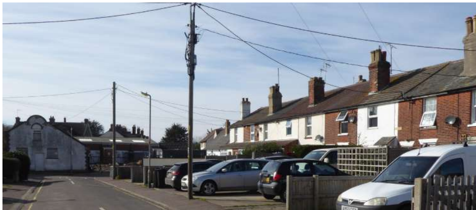
Figure 90 Images above: views of Alfred Terrace
