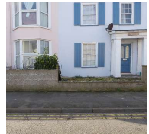
Figure 97 Example of boundary wall replacement
