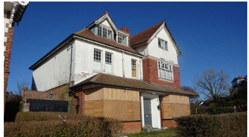
Figure 103 Vacant building on Frinton's Esplanade
