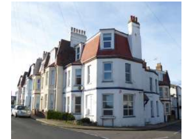
Figure 64 Large corner building
