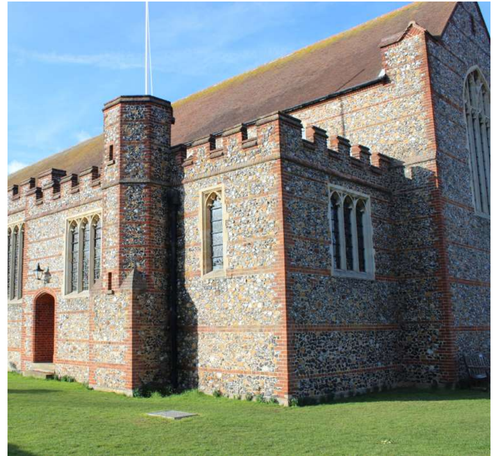
Figure 33 St Mary's Parish Church
