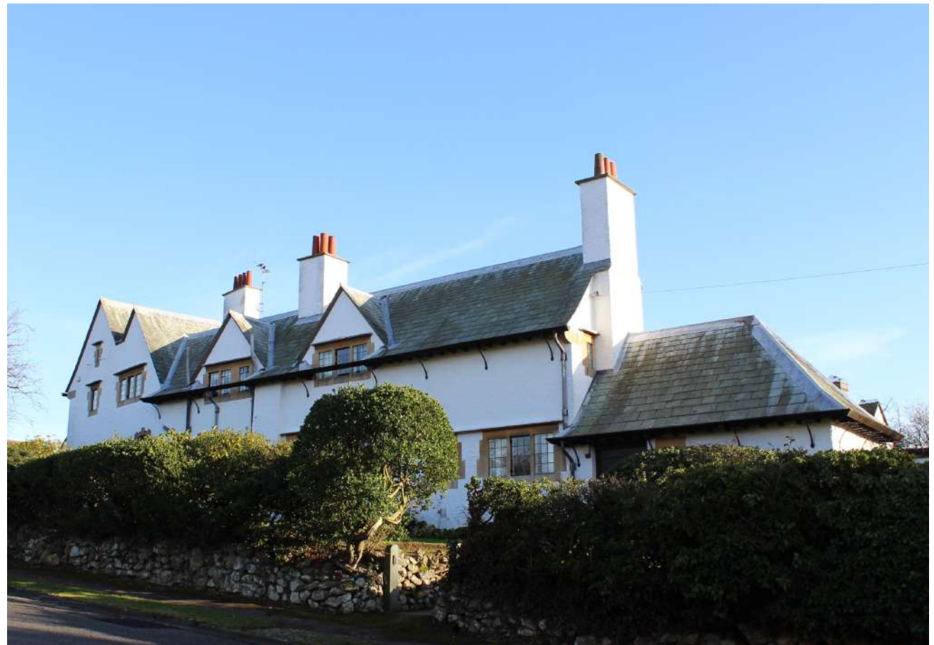
Figure 29 The Grade II Listed Homestead
