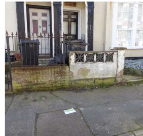
Figure 96 Example of boundary wall
