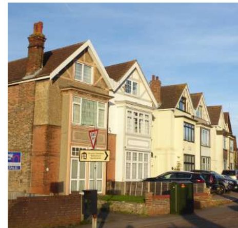
Figure 81 Terraced row of residential dwellings
