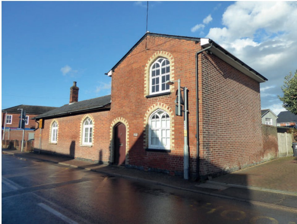
Figure 26 Photograph of Old Hall Cottage
