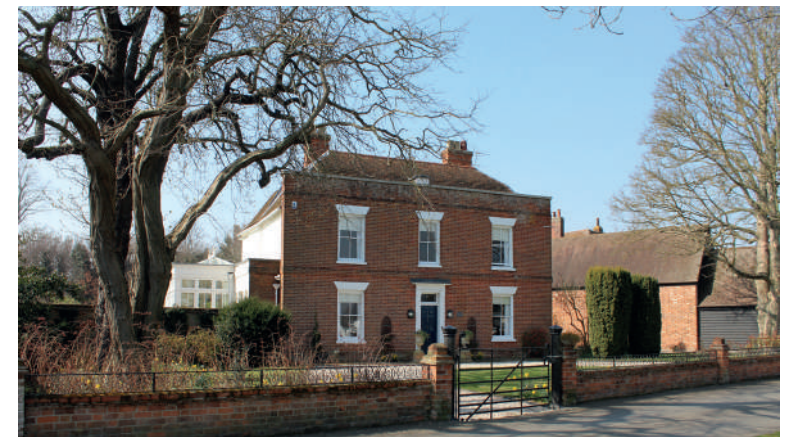
Figure 15 Photograph of The Old Rectory
