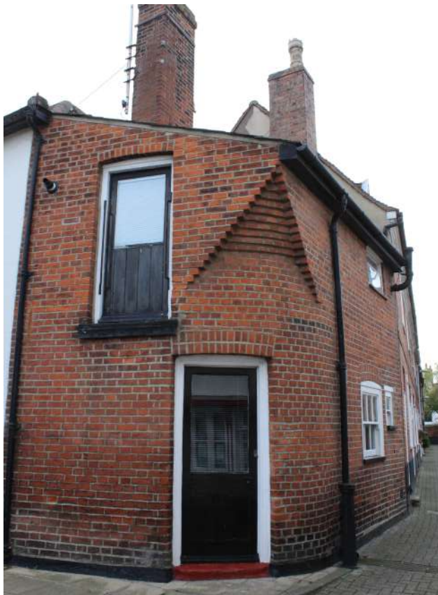
Figure 37 Building detail on George Street
