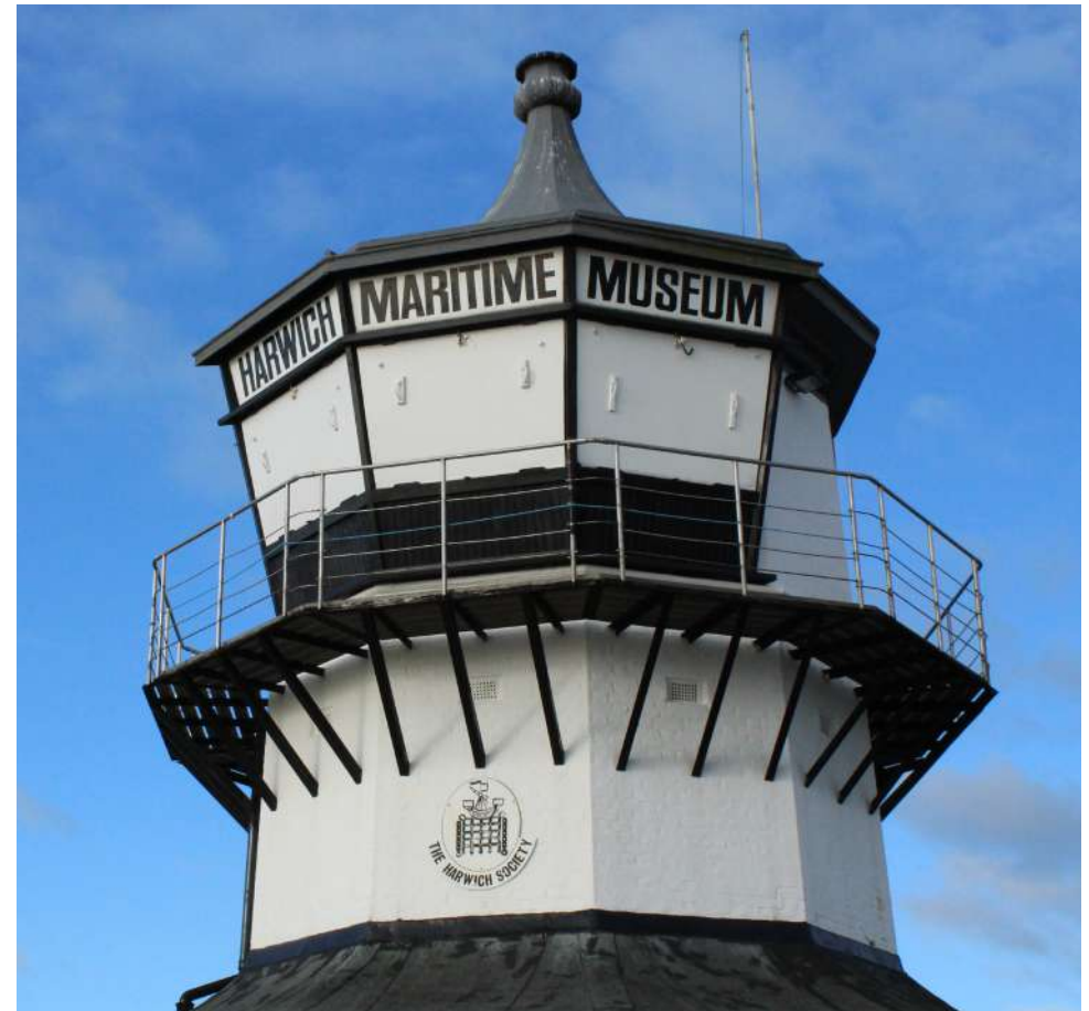
Figure 44 Harwich Low Lighthouse
