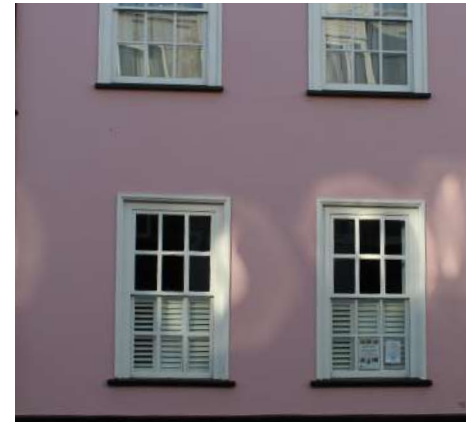
Figure 16 Example of Georgian facade
