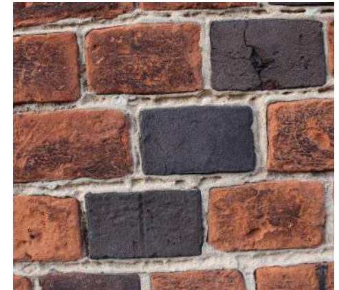
Figure 17 Red brick within the Conservation Area
