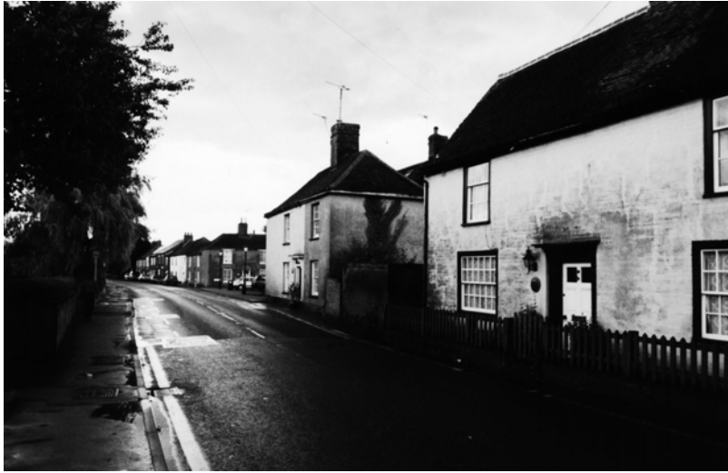
1. The High Street looking north eastwards, with the island block on the right. The strong visual effect created by the historic buildings lining the main road is diminished by the corridor-like appearance of the High Street. Improvements could be considered to the surface both of the carriageway and the footpath.
