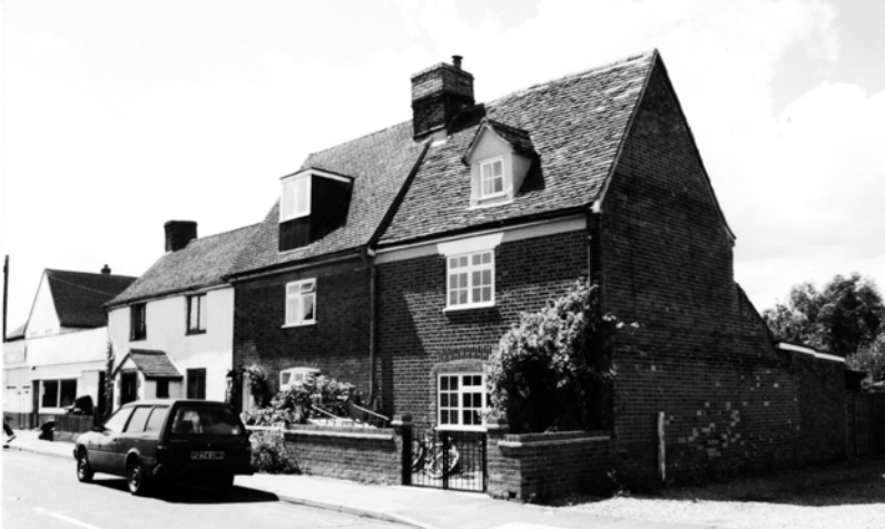
6. Vine Cottage and its neighbour are attractive vernacular buildings at the south western end of the Area. Both have been the subject of minor alterations which affect their historic character: Readily apparent are the modern dormer to the Vine Cottage and the modern windows to No 1.
