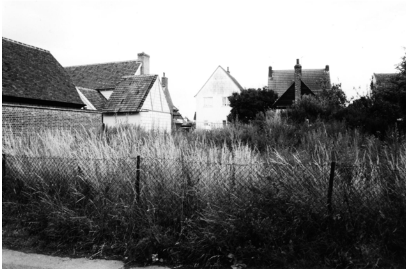
9. The vacant plot in the centre of the Area, seen from Queen Street. Of significance are the simple detailing of visible buildings, and the importance of roof design and materials in this village setting.
