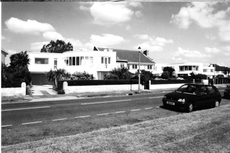
4. Two Estate houses and the former Estate Office at the far right make an impressive group on Cliff Way, interrupted only by the well considered post-war design, which must however be considered as a neutral feature in this special context.
