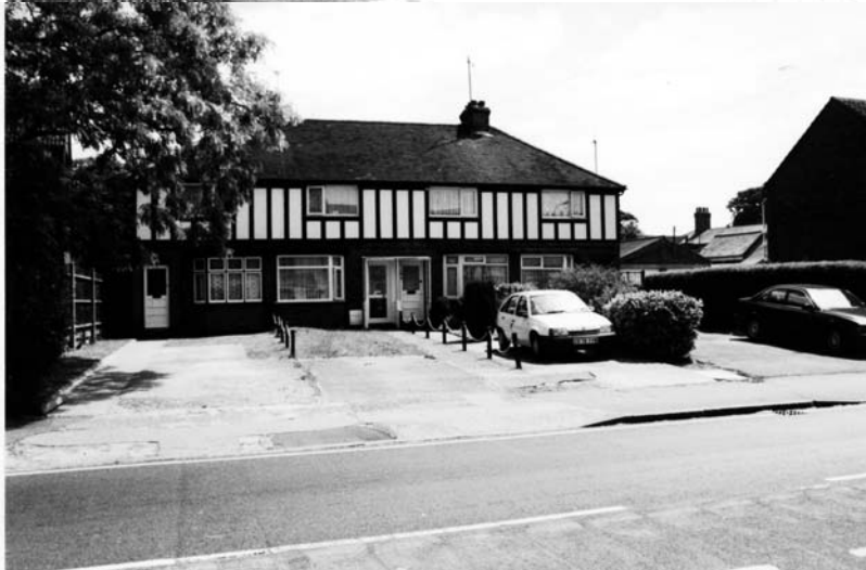
4. These properties on North Road make very little contribution to the Area, which recognises the commercial centre of this old village. The matter has not been helped by the loss of the front garden boundaries as a result of vehicle parking.
