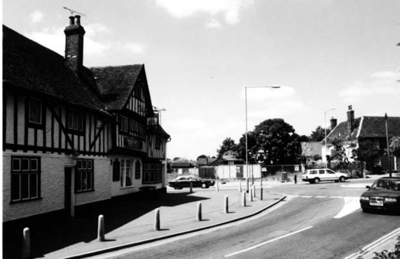
11. Once again, the demands of vehicular traffic have compromised the setting of the Ship Inn and its neighbouring Listed Buildings. The forecourt to the Ship is particularly plain and could do with visual improvement.
