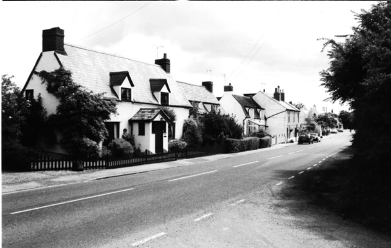
7. Another development form of great significance is exemplified by this group of cottages with varied relationships with the main road. They gain consistency from the limited range of facing materials, though the variety of garden frontage styles is a modern phenomenon. Gable treatments become extremely important visually.
