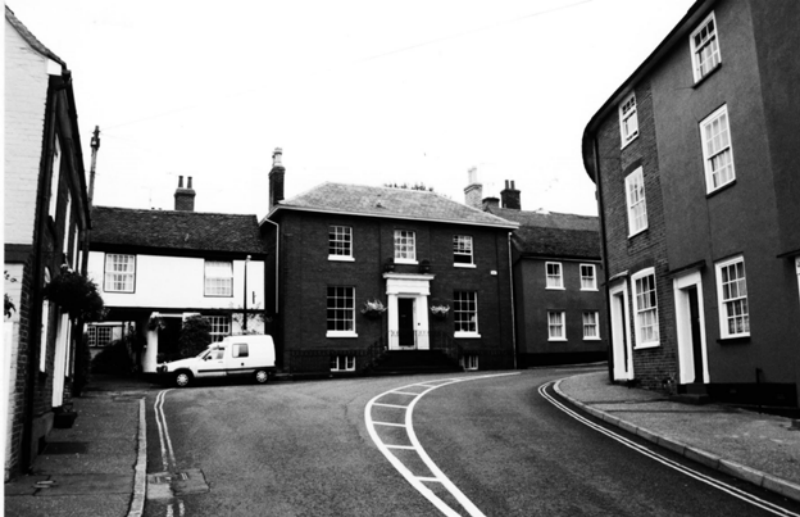
1. The entrance to Manningtree's High Street from the town. One of the most impressive sequences in the town. Victorian and "polite" houses all have a strong relationship with the street and with each other.
