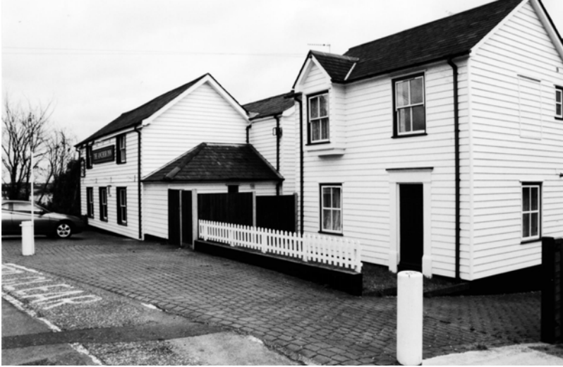
22. The Anchor Inn and the new house next door are maintained under their weatherboarded facades. The replacement of the chimneys to the original building is regrettable, and the printed concrete forecourt has an insistent quality not shared by its relative openness to the street.
