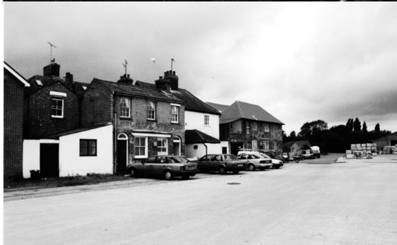
16. Varied developments to the north of Fountain Street look out over the Stour estuary. The wide quayside is a thoroughly industrial location. The building in the distance is that which detracts from the setting of the Towers.
