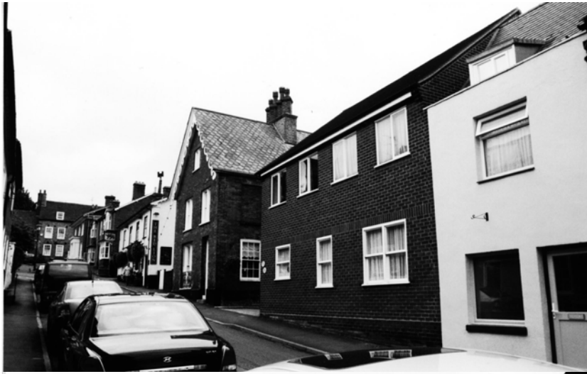
5. South Street climbs away from the medieval town. Development beyond Stour Street is more varied, including the delightful incident of the substantial gable pictured here, as well as the uninspiring post-war example to the right.
