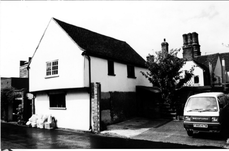
3. Stour Street to the rear of High Street contains a number of properties. This particular example demonstrates the development of a whole medieval burgage plot. Some modern developments are less sympathetic, and the parking areas are handled in a variety of ways.
