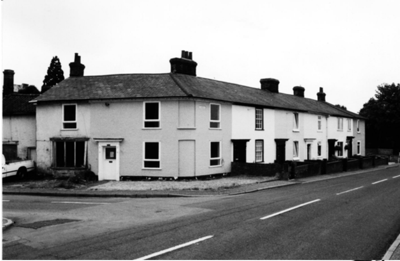
21. James Terrace at the eastern end of High Street is a significant part of the development history of Mistley. Though it retains its slate roof and door cases, the terrace has lost all its original window details, a particular problem given its prominent setting.
