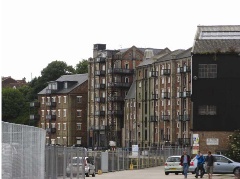
Quayside fence at Mistley
