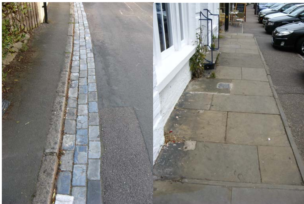
Distinctive blue-glazed bricks form a gully next to a line of granite kerbs.
