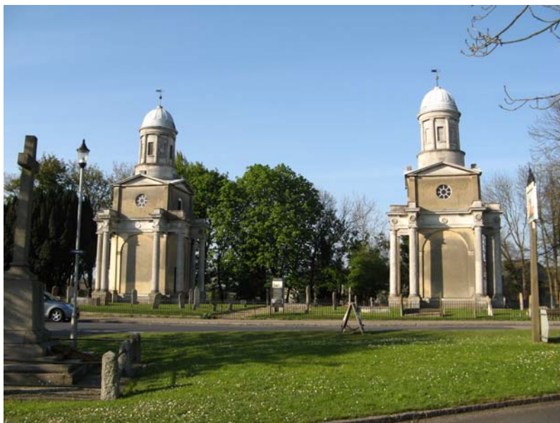
The Mistley Towers – Designed by Robert Adam in 1735 for a church that was demolished in the 1860s
