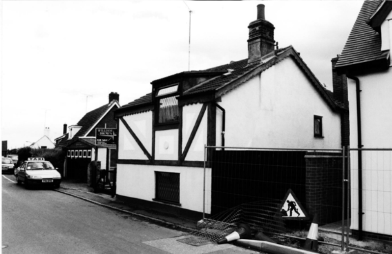
11. Rose Cottage is evidently of some historic interest but this is overlain by the modern finishes which clash with the limited palette and neighbourly qualities of most other older buildings in the Area. Its garage is not of traditional construction and is unfortunately prominent in the street scene.
