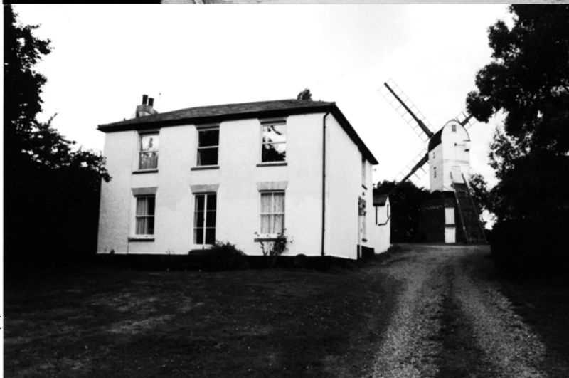
4. While the Mill is an important part of the local landscape it is less visible from the village until approached from T. Street. The Mill, its house, outbuildings and the drive itself make a fascinating group, which would be enhanced by improvements where possible to the less attractive parts of the compound.
