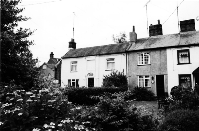
8. This row of cottages has a different relationship to The Street from most older properties in the Area. The essential enclosure and character of the Area is maintained by their continuous frontages and in the way these front gardens contrast with frontage buildings and enhance the visual quality of the village
