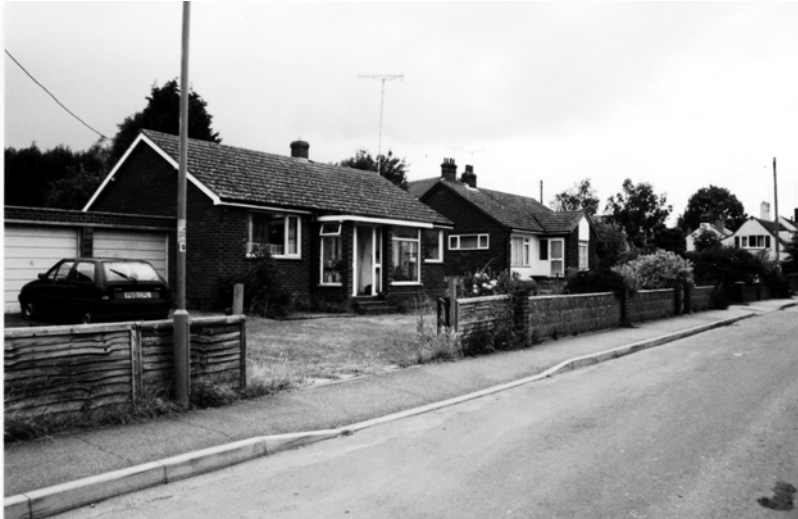
9. These post-war bungalows fronting The Street must regrettably be regarded as negative features because their siting and built form do not reflect the characteristics of the surroundings. The front gardens and walls are also visually disappointing and are suggested for enhancement in the report.
