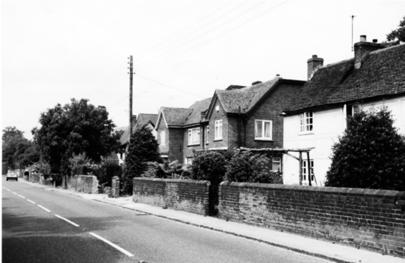
5. Houses of various ages come together behind a continuous brick frontage wall to provide the most consistent street scene in the Area. The quality of this part of the Area is dependent upon the continued maintenance of properties and front gardens alike.
