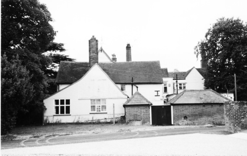
2. Tendring Hall seen from the drive to the north. While the main façade of the Hall has a formal setting, the side elevation and its attendant outbuildings form an interesting sequence of spaces, framed by mature trees and affording views over open countryside.
