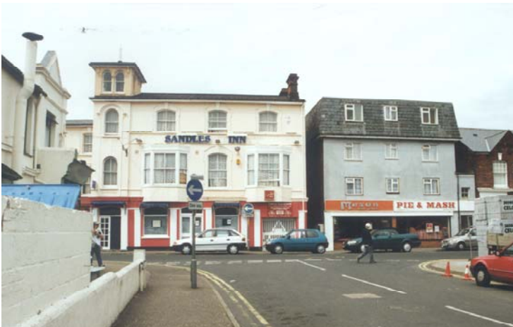
10. The Sandles Inn on Rosemary Road is prominent on the previous view from Orwell Road. Closer to its sash windows, projecting bays and its tiny belvedere can be appreciated. Less happy is the unfortunate building to the right, the lowest-common-denominator-design of which is a negative feature in the street scene.
