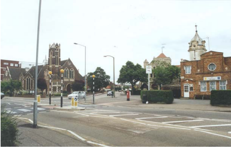
13. Public buildings surround the junction between Holland Road and Carnarvon Road. This important location is let down by the dominance of road considerations and the bleakness of the surrounding pavements. The trees are particularly important, but the area needs comprehensive consideration.
