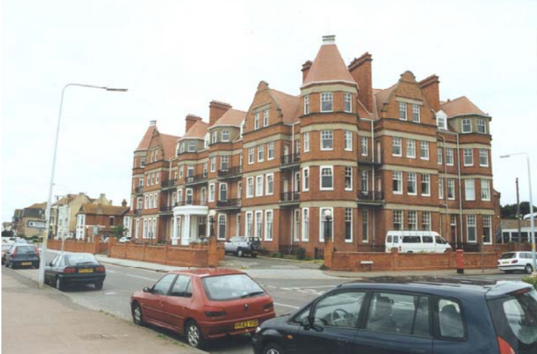
16. The former Grand Hotel of 1892-97 by Gale and Farthing of Smith Son and Gale has limited decorative appeal: its importance is as the earliest use yet known of a completed and coherent structural steel systems. It is extremely prominent in longer seafront views and is with the Towers a sensible termination to the Conservation Area.
