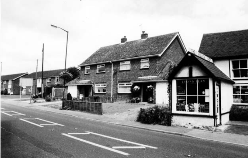
10. While The Village Shop is an important part of the character of the Colchester Road, beyond its distinctive projecting shop front stand a pair of uninspiring post-war houses which are recommended to be excluded from the Area.
