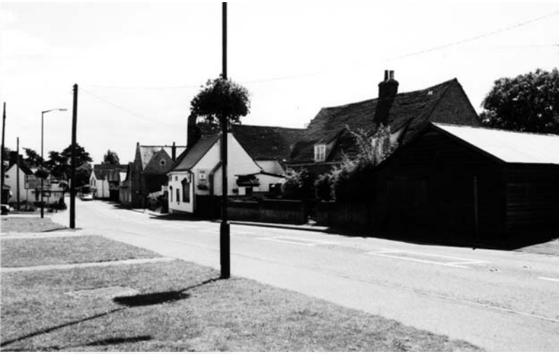
5. The approach to the Area along Colchester Road from the west. The large and simply-detailed timber shed on the right is a prominent feature, and relates well to the surrounding vernacular architecture .
