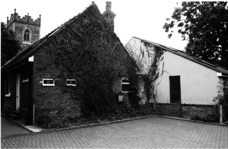
9. These office conversions front the car park and access to the surgery on The Street. Side and rear elevations in older villages settings often require more careful consideration given the generally informal character of building and property layouts.
