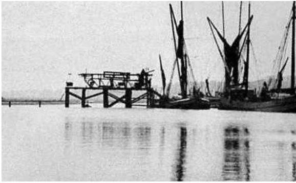
Sand and gravel being loaded onto sailing barges in Alresford Creek
