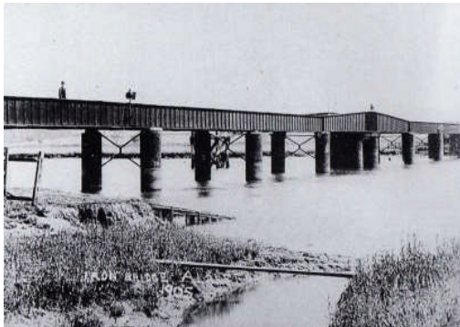
Iron Swing Bridge (Picture c.1905)
