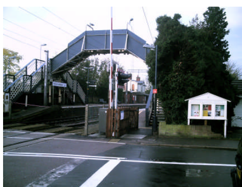
Alresford Station with automatic gate
