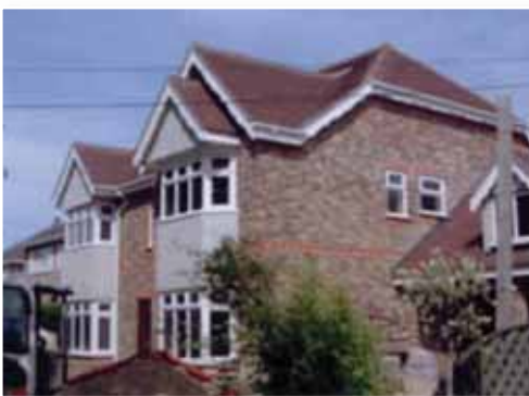
Infill building on Clacton Road. An example of a house which fulfils all the criteria as set down in Policy RA4
