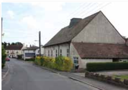
Village Hall exterior
