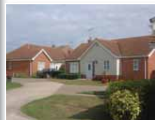
Manor Court, Manor Road Built in late 2000
