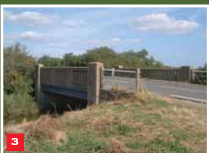
3 Exit Bridge to Clacton over Holland Brook
