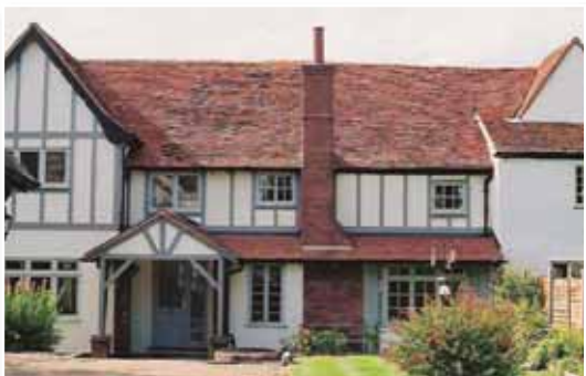
Ring cottage, Little Clacton Road 16th/17th century with 20th century alterations and additions. Timber framed and plastered. Red plain tiled roof
