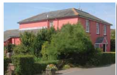
Anne's cottage. Church Lane. Retained details make a major contribution to character.
