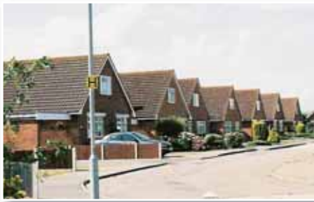
Laxton Grove and Orchard Drive built in the 1970's and 80's a development of approximately 60 properties
