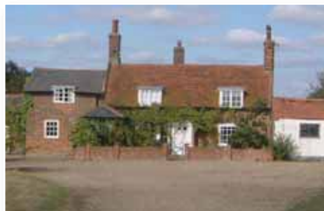
Geat Holland Mill House, Little Clacton Road. 19th century red brick. Red plain tiled gambrel roof. Extended to former granary with grey slate roof
