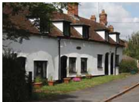
Tudor Cottages, Rectory Road. Row of 16th century cottages. Timber framed, brick façade now rough rendered (1720 – 1730)
