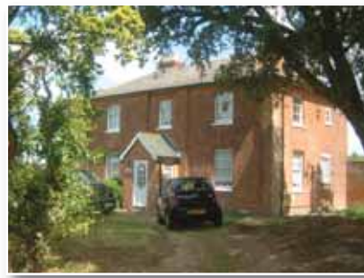
Larges Farm Rectory Road. A former farm house in traditional red brick under a slate roof Note new porch in keeping with style and materials
